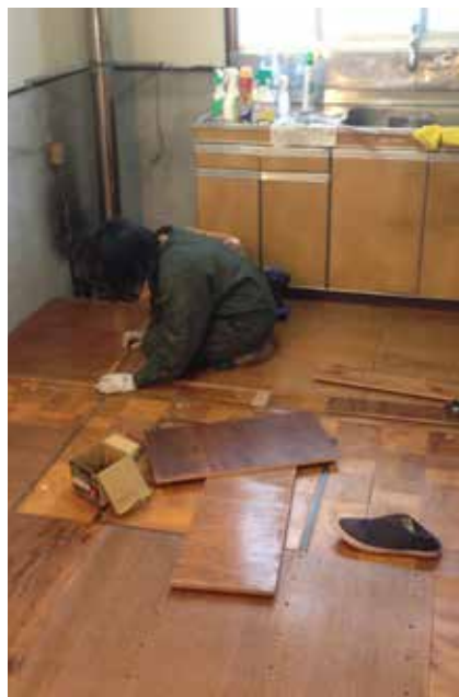
Installing a new layer of flooring on top of the old one in the kitchen.
