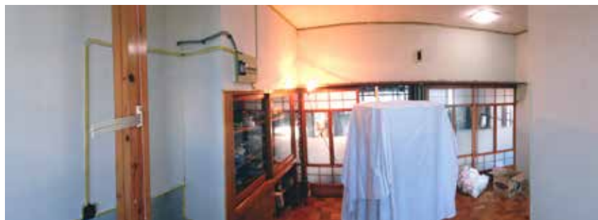
Giving the kitchen a new coat of paint.
