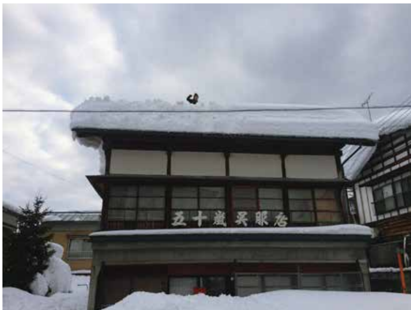
Cleaning snow off of the roof this winter.
