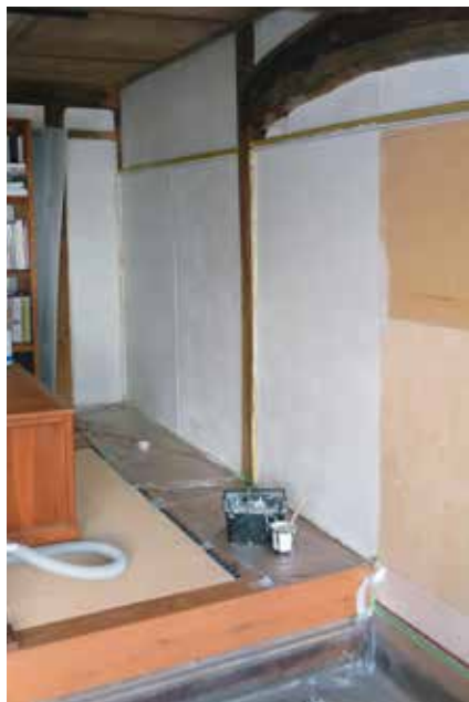
Putting up new walls in the community space.
