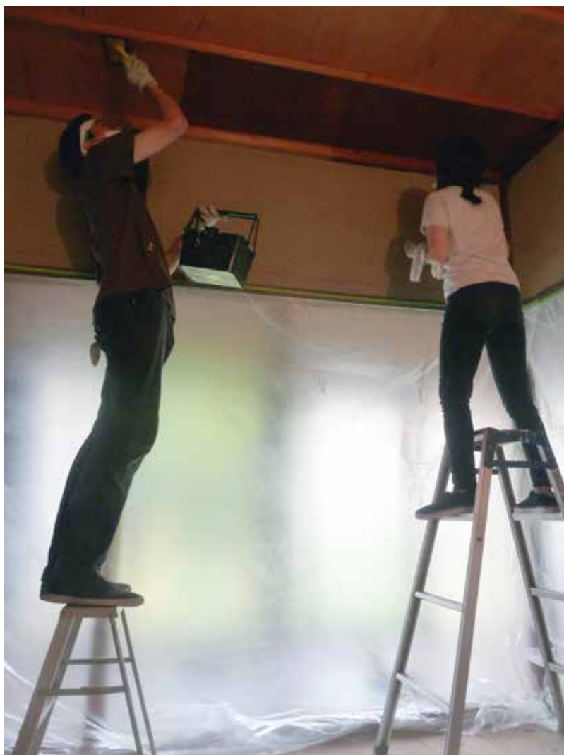
Staining the ceiling in our studio and living room.
